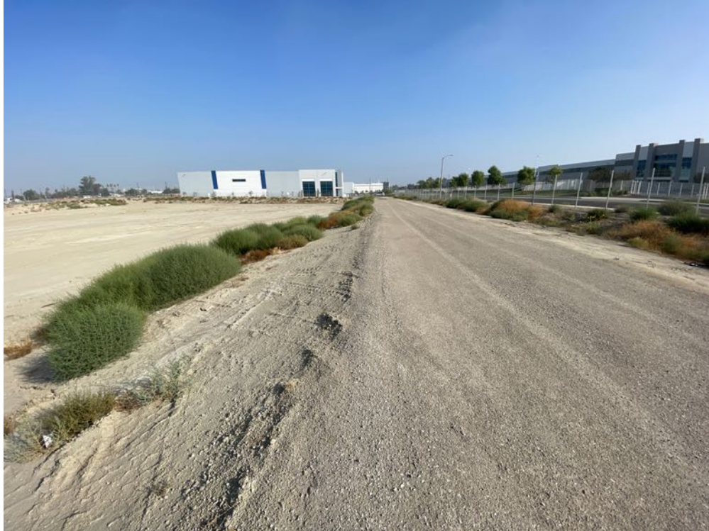
Photo 3. View of a developed roadway around a disturbed basin, facing north.
